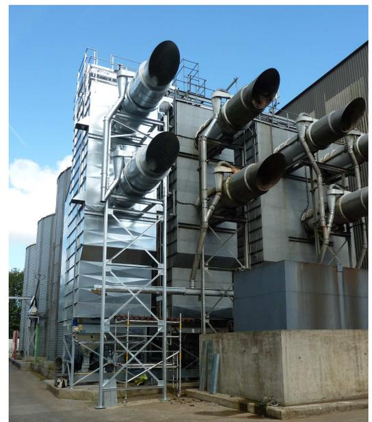
Turboclean units on a Svegma Grain Dryer.
